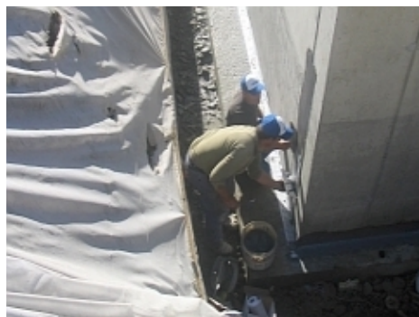
Application of VANDEX CONSTRUCTION JOINT TAPE on horizontal joints
