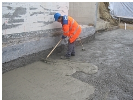
Application of VANDEX UNI MORTAR 2 on to the blinding concrete
