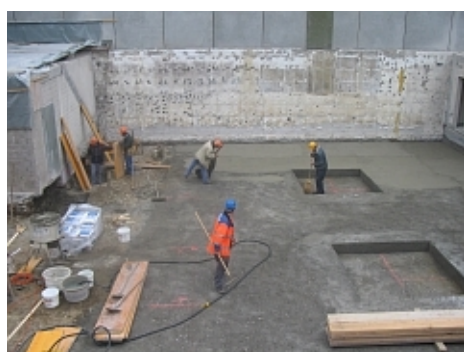
Waterproofing under the foundation with VANDEX UNI MORTAR 2
