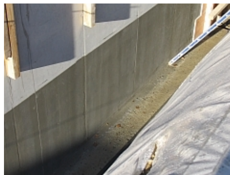
Waterproofing with VANDEX CEMELAST
