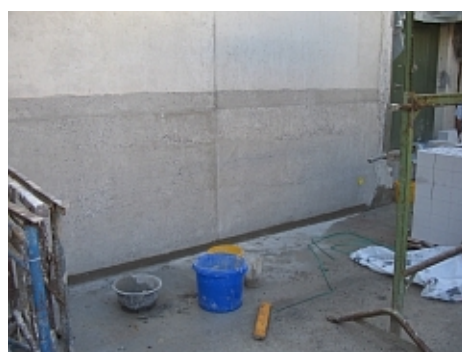
Prepared surface for the application of VANDEX CEMELAST
