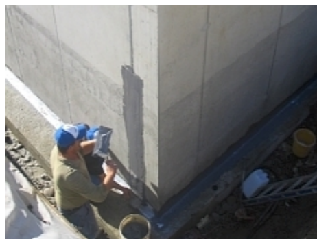
Application of VANDEX CONSTRUCTION JOINT TAPE on vertical joints
