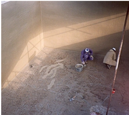
Preparatory work on base slab using VANDEX UNI MORTAR 1 Z
