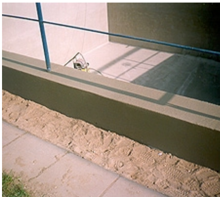
Parapet walls treated with VANDEX CRS OS 95, 3.6 kg/m 2 (2 mm)
