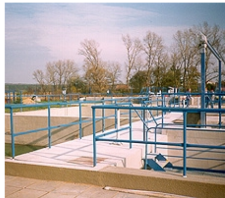
Finished overview of renovated sewage treatment plant
