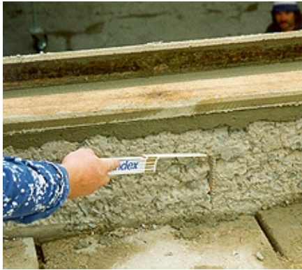
Concrete repair work using VANDEX CRS REPAIR MORTAR 05
