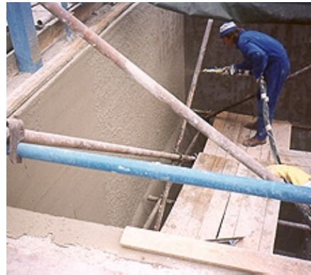
Spraying VANDEX UNI MORTAR 1 Z, 16 kg/m 2 (8 mm)
