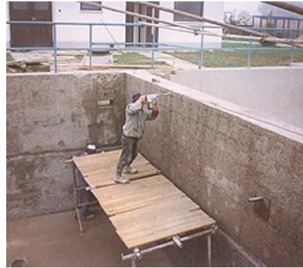
Preparatory work of walls after high pressure water jetting
