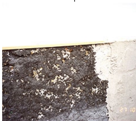
VANDEX ROUGH CAST on the left and VANDEX REFURBISHMENT PLASTER white on the right
