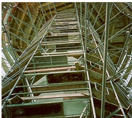
Scaffold around the tower
