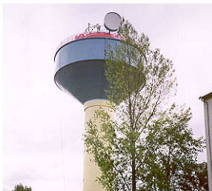
View of the finished refurbished watertower
