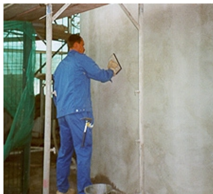
Finishing of VANDEX CRS LEVELLING COMPOUND LC
