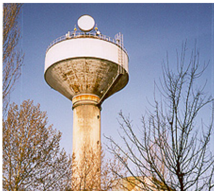
The tower before the start of the refurbishment work
