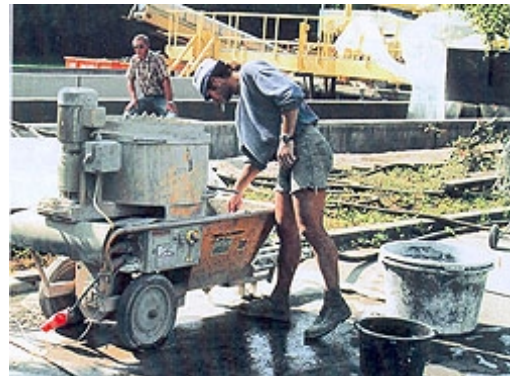
Preparation for the spray application Sewage plant prior to refurbishment
