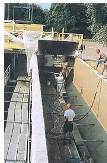
Application of the protective coating
