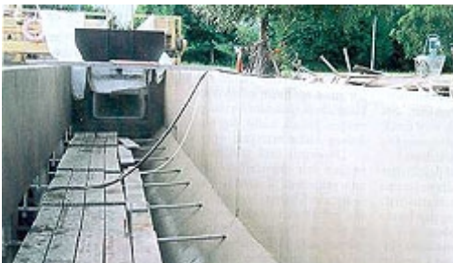
Treated areas before curing measures
