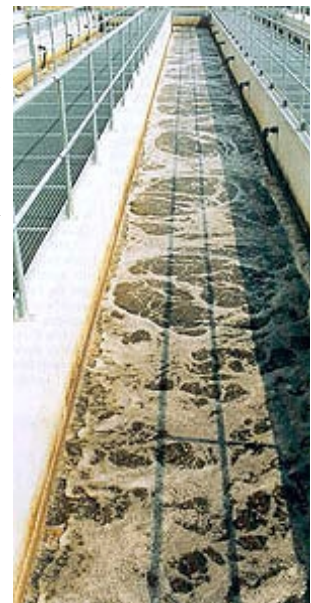
Refurbishment with polymer modified mortar completed: the aeration tank is in operation
