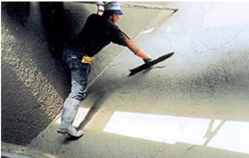
Levelling the freshly applied mortar coating
