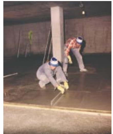
Figure 2: Levelling and providing a slope with steel rails.
