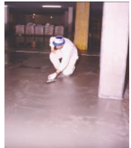
Figure 3: Trowelling the screed to a smooth and dense surface.
